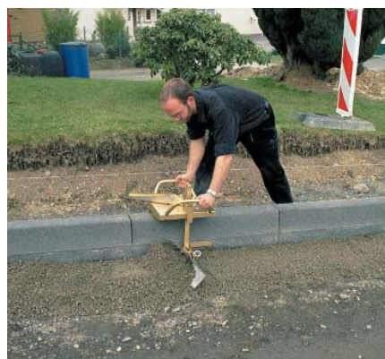
The device is pushed by the operator. Large rollers rolling on top and on the rear side of the kerb take off the reference height and transfer it to the plowshare.
